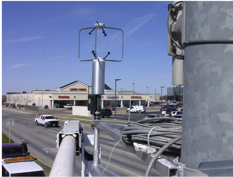
Figure 4.7: Ultrasonic anemometer attached to the pole
