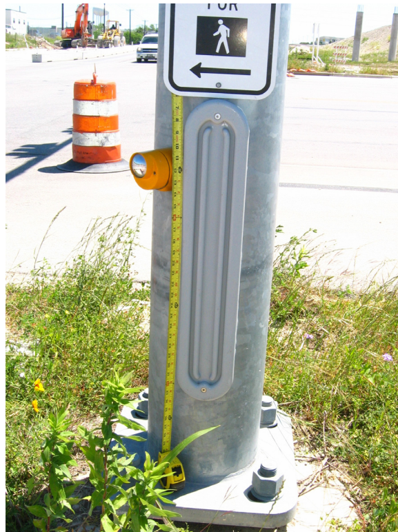
Figure 5.2: A handhole is typically cut out of the steel pipe near the base of the pole
