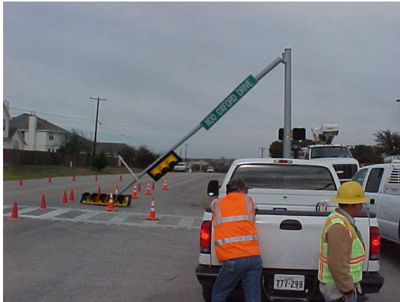
Figure 4.10: Failure of traffic signal structure in Pflugerville in December 2003
