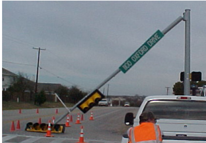
Figure 1.1: Failure of traffic signal structure in Pflugerville
