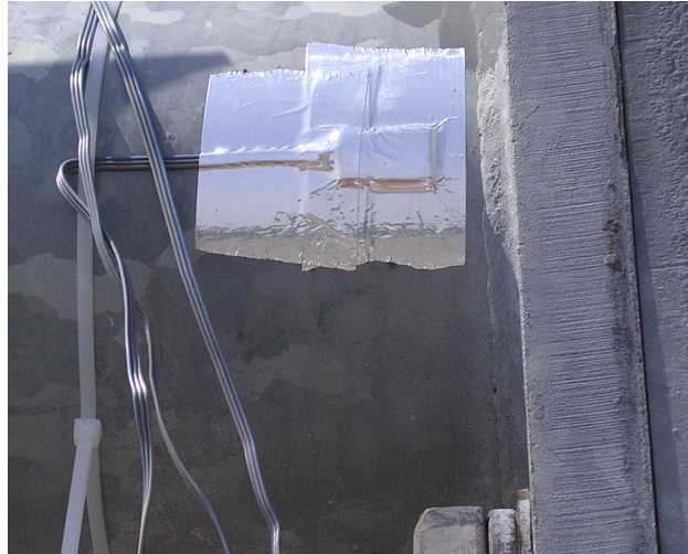
Figure 4.4: Strain gauge attached to mast arm and weatherproofed
