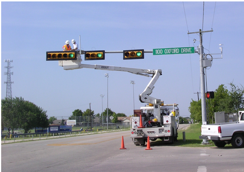
Figure 4.13: A bucket truck is utilized to pluck the structure
