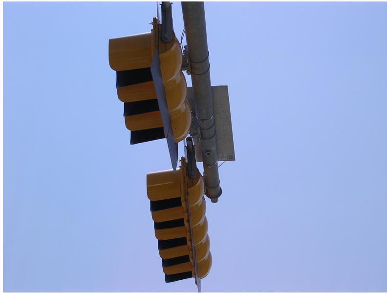
Figure 4.12: The traffic signals have rounded backs and are below the mast arm
