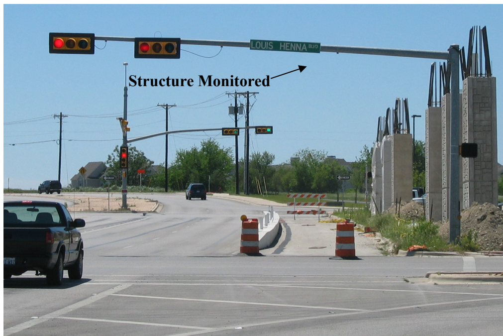
Figure 4.36: Traffic signal structure monitored in Round Rock
